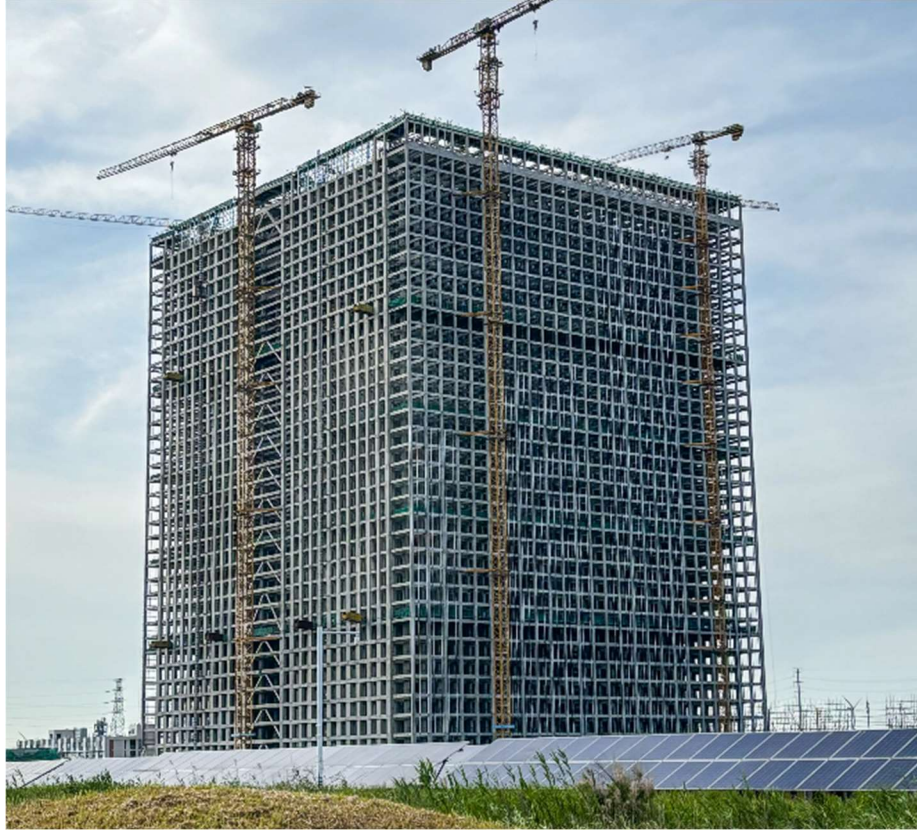
Figure 2.7 Rudong Energy Vault Evx 100 MWh commercial unit
