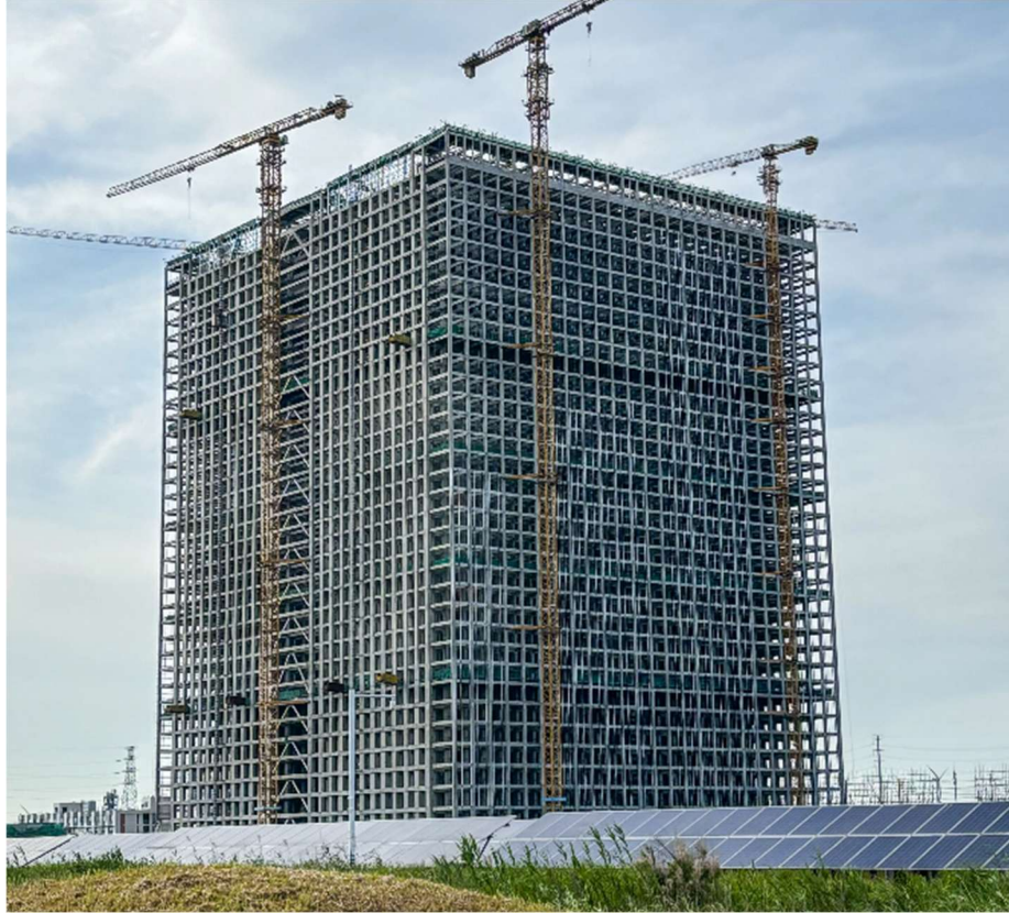
Figure 2.7 Rudong Energy Vault Evx 100 MWh commercial unit
