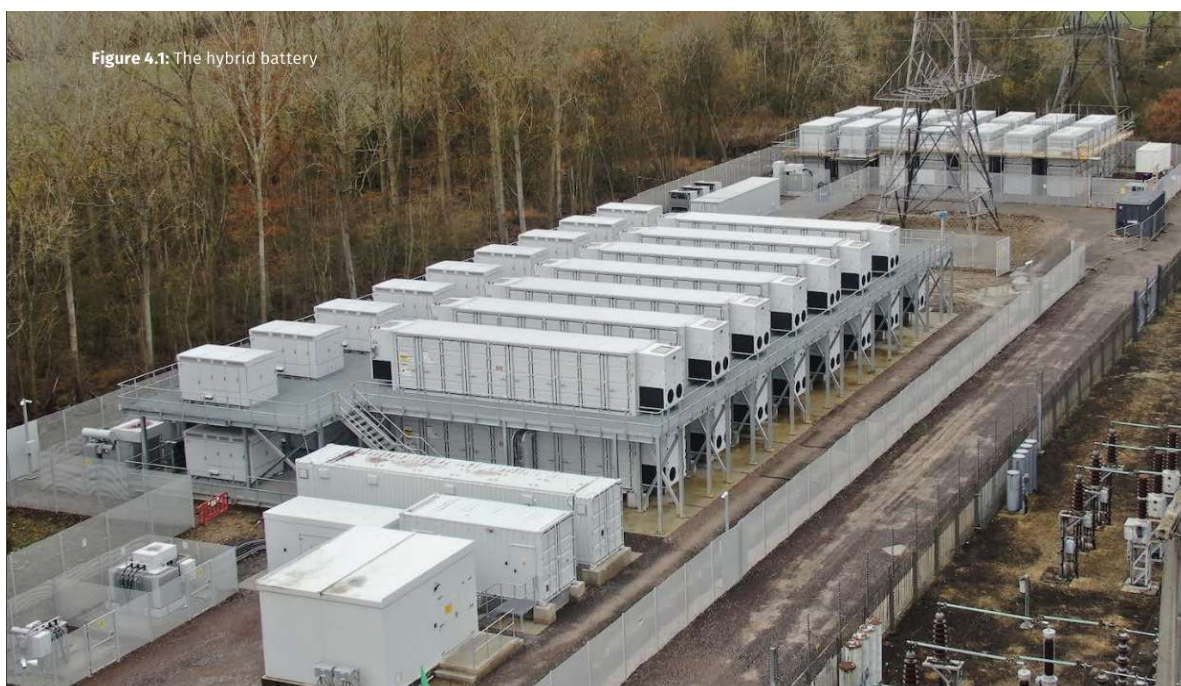
Figure 8.23 - The hybrid battery consists of two core assets, a 50 MW (peak power) / 50 MWh (energy) lithium-ion battery and a 2 MW (power) / 5 MWh (energy) vanadium redox flow battery.
