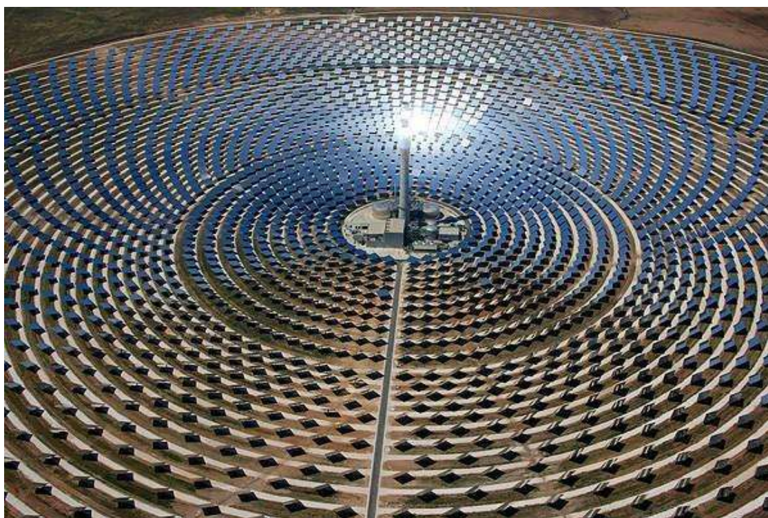
Figure 11.2 Gemasolar Concentrated Solar Power, Seville
