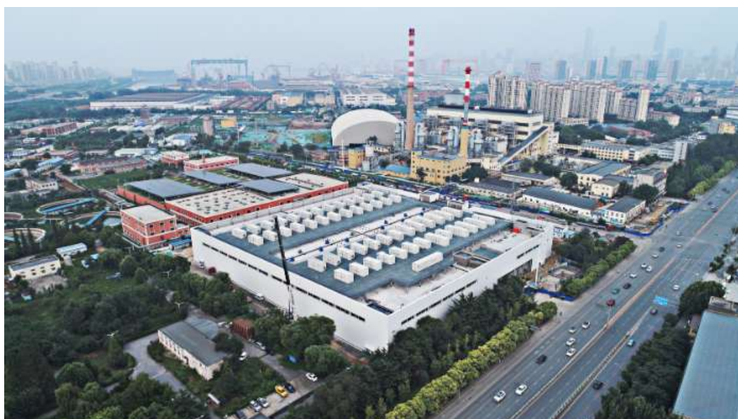
Figure 8.19 – Dalian Flow Battery Energy Storage Peak-shaving Power Station 305
